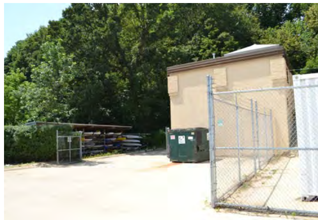
Existing Sanitary Pumping Station
